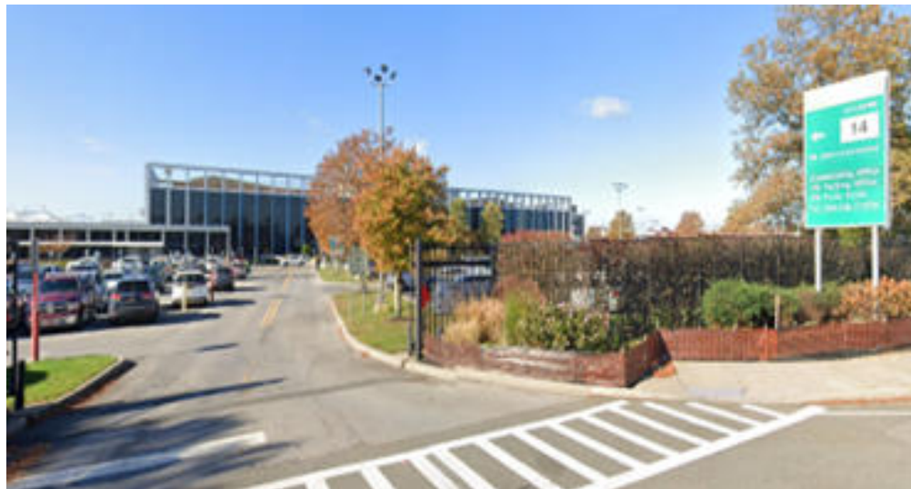
PANYNJ - JFK Administration Building #14, NY
